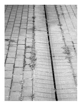
Plants in mortar joints on Cromwell Highwalk
