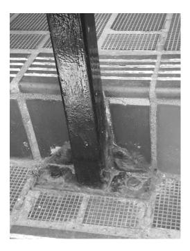
Corroded fixings on steps up to Beech Highwalk from Lauderdale Place
